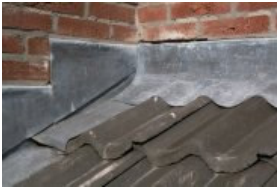
Application of lead on roofs.
